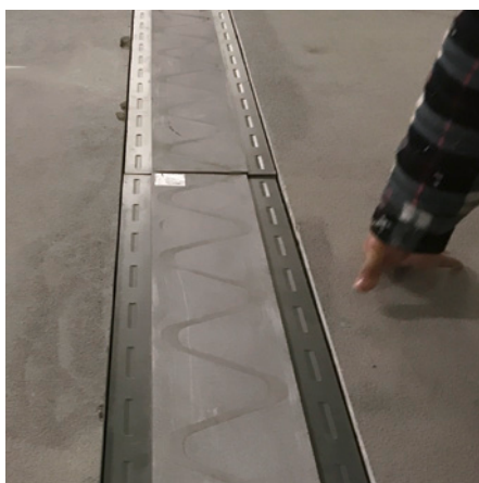
Installing the joint connection profile MC-Floor Connect CP
