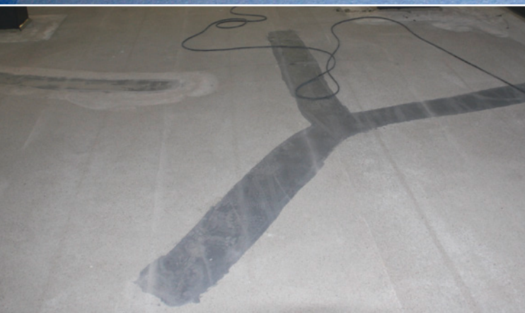
Crack patch prior to top-coating
