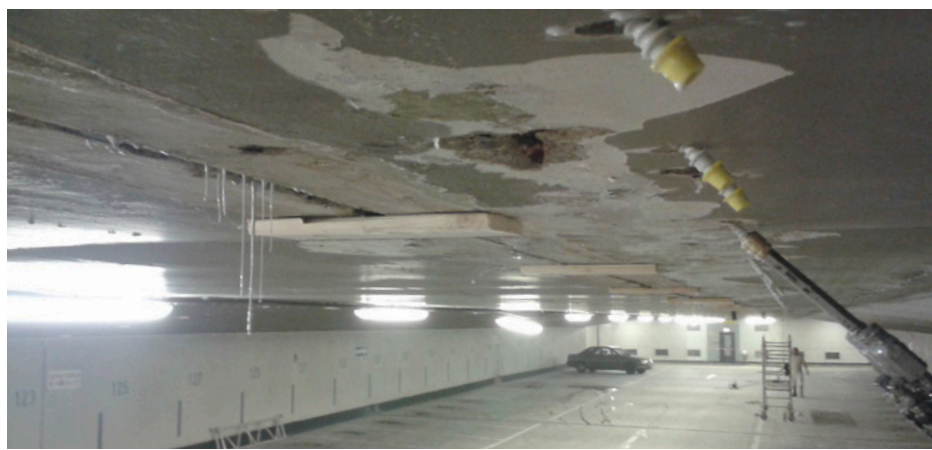
Injection of the deck joints
